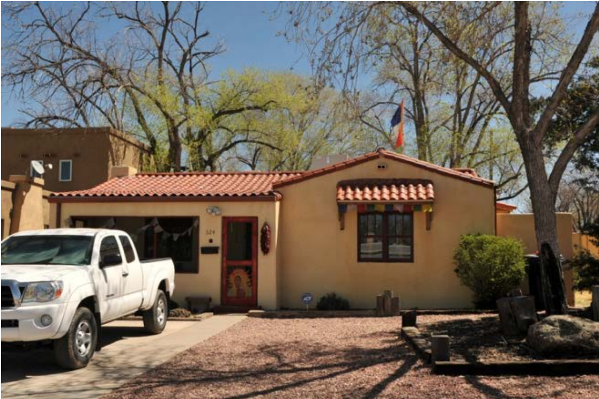
Figure AB-1 – Photograph of the residential structure in Albuquerque, New Mexico
